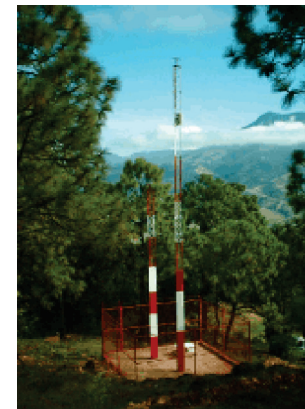
Typical Seismic-Sense Station
